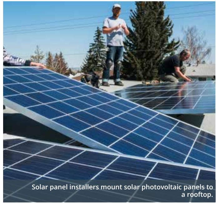
A solar panel technician outfits a panel prior to installation.
