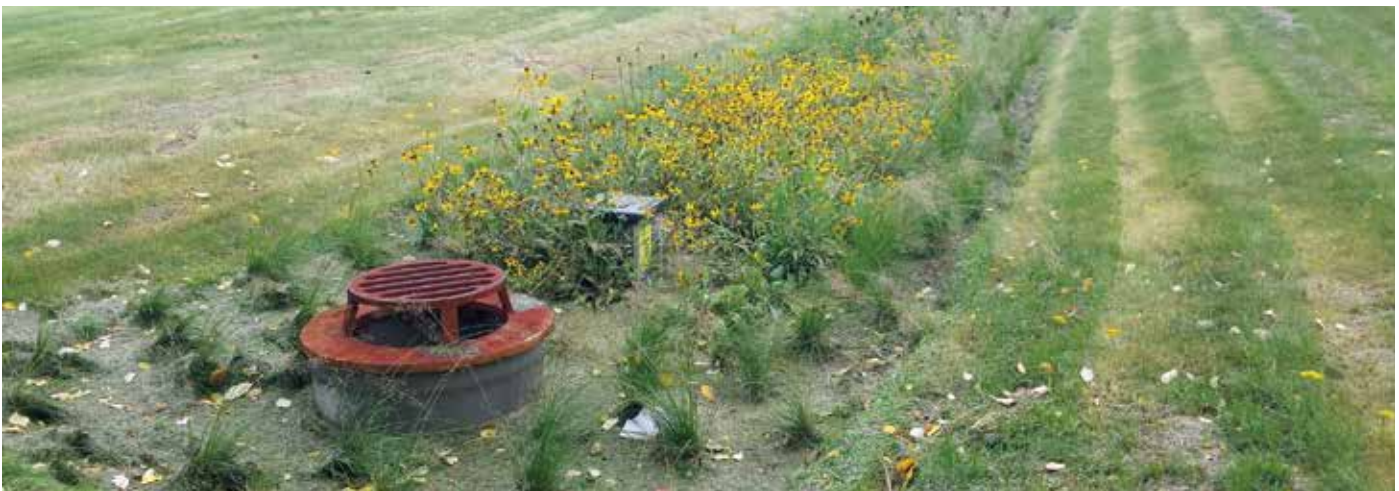
Bioswales capture and treat pollutants in stormwater runoff before the water reenters streams and rivers. Bioswale installation can be partially reimbursed through the City's Stormwater BMPs Cost-Share Program.
